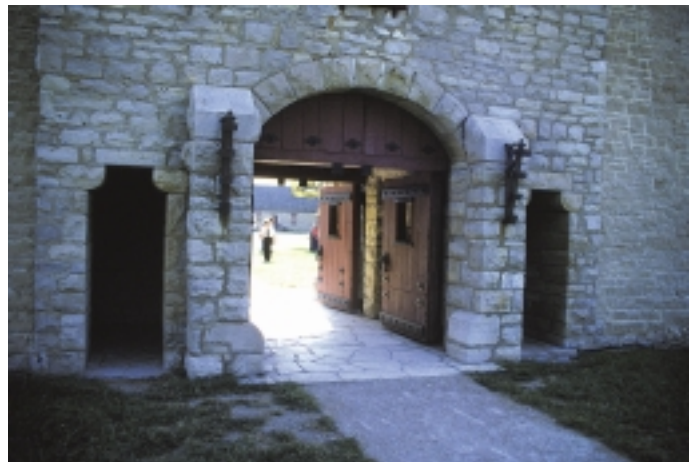
Reconstructed main gate, Fort de Chartres, Randolph County, Illinois. Courtesy of Gary Andrashko, Illinois State Museum.
